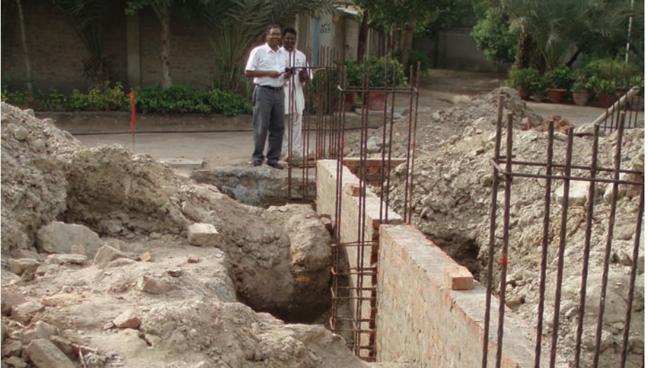
Rebuilding the laundry
