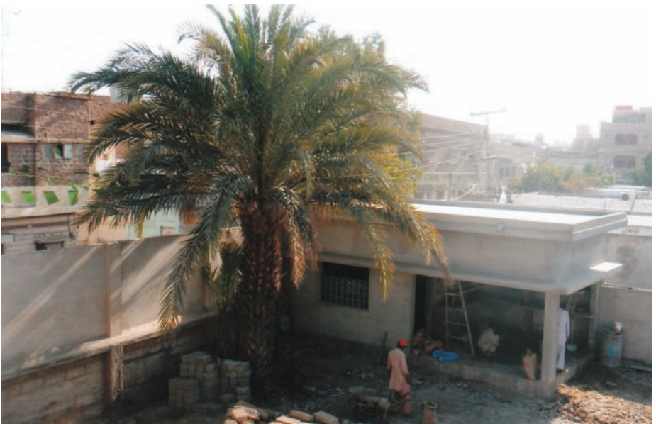
The nearly completed laundry
