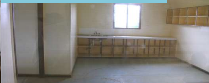
Komo hospital ward room
